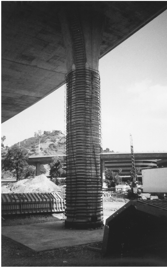
FIGURE 8.6 Reinforcement confinement retrofit.
