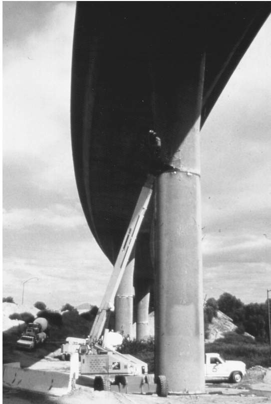
FIGURE 8.8 Steel jacket column retrofit.
