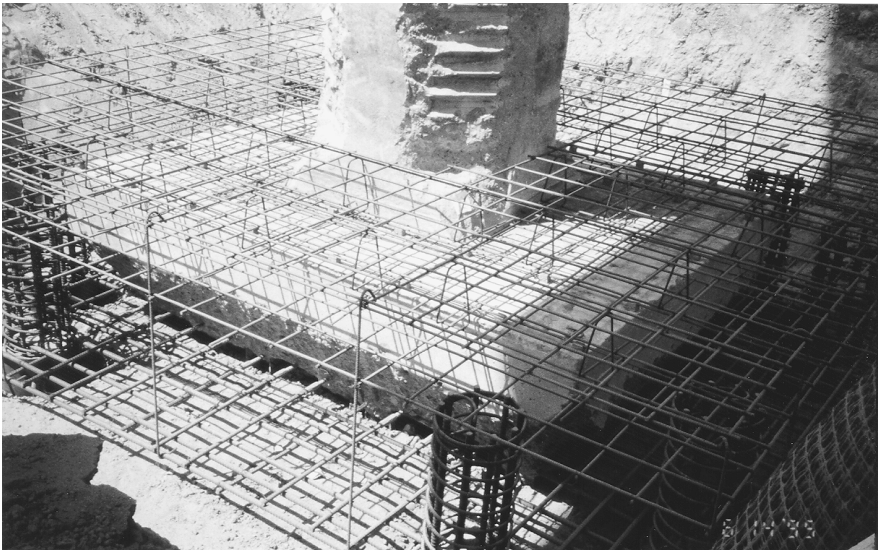
FIGURE 8.16 Typical footing and pile cap modification.
