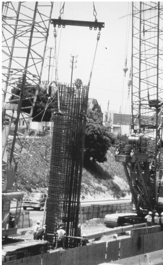
FIGURE 8.11 Column-reinforcing steel cage.
