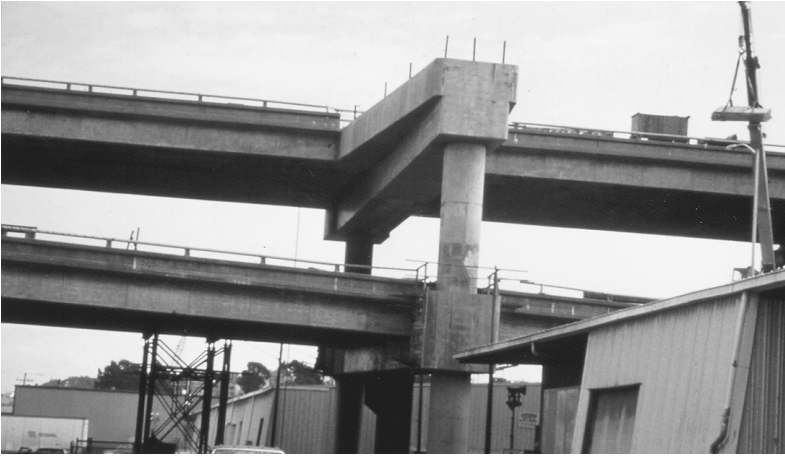
FIGURE 8.14 Completed retrofitted structures.
