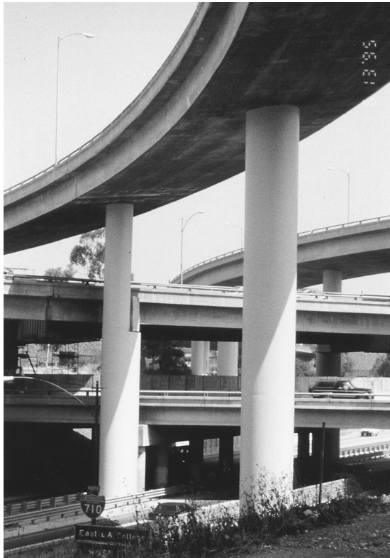
FIGURE 8.17 Completed seismic retrofit of I-5/710 interchange in Los Angeles.
