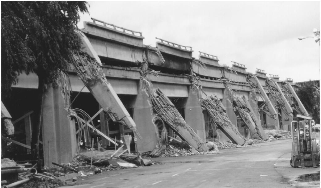
FIGURE 2.29 Cypress Street Viaduct collapse in the 1989 Loma Prieta earthquake.
