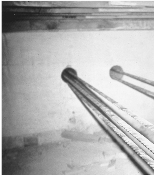
FIGURE 8.3 Hinge joint restrainer.
