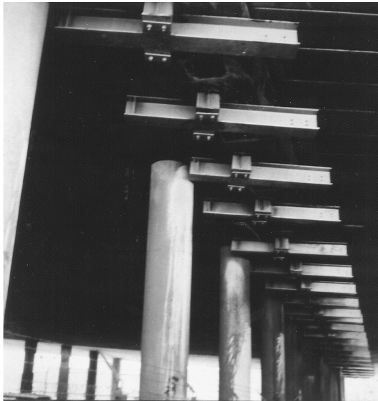
FIGURE 8.5 External hinge extenders on Santa Monica Freeway structures.
