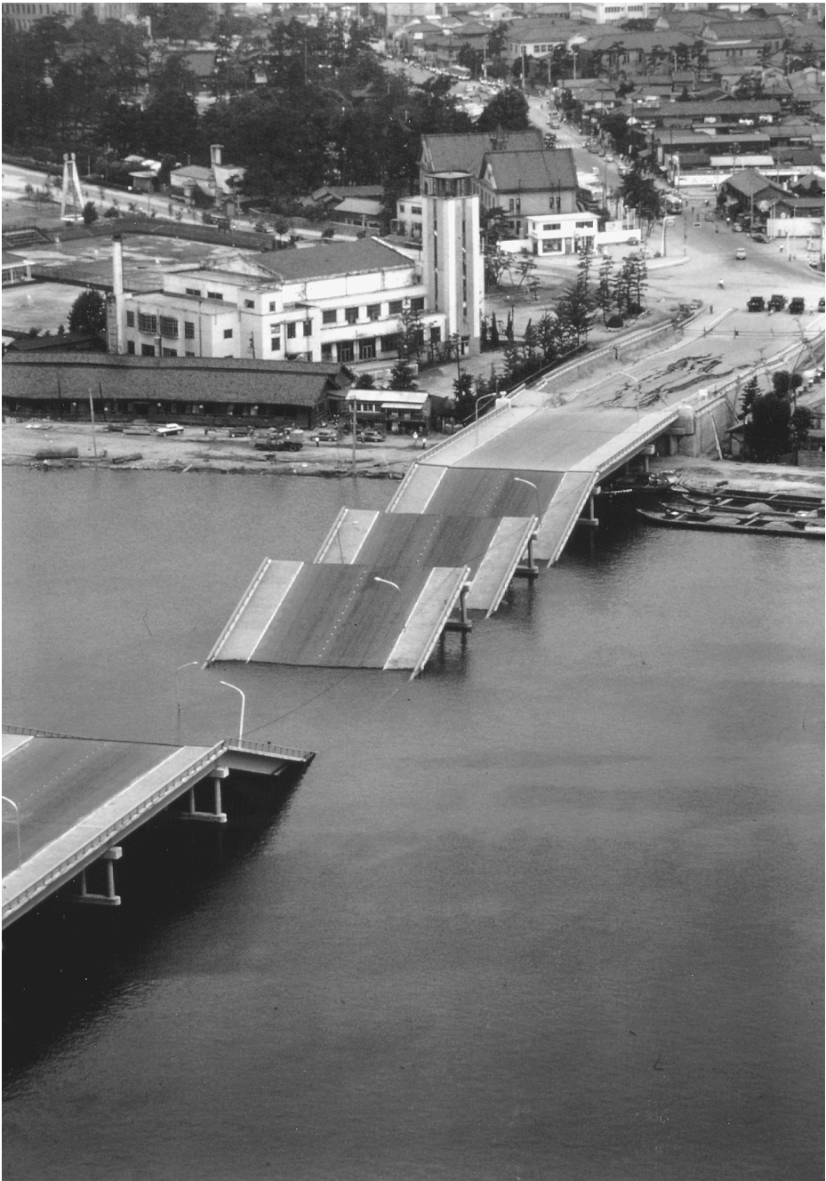
FIGURE 2.8 Showa Bridge collapse in 1964 Niigata earthquake.
