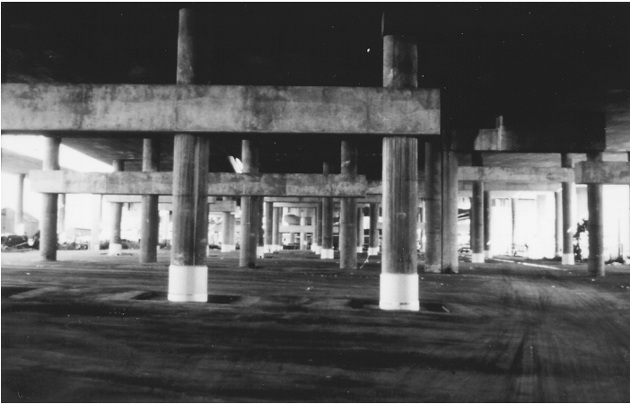
FIGURE 8.10 Steel jackets and bond beam — Santa Monica Freeway.
